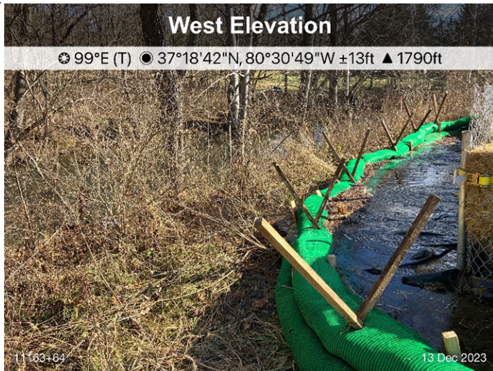
Figure 3: Sta 11163+64, dewatering structure in place and functioning for S-NN17.
