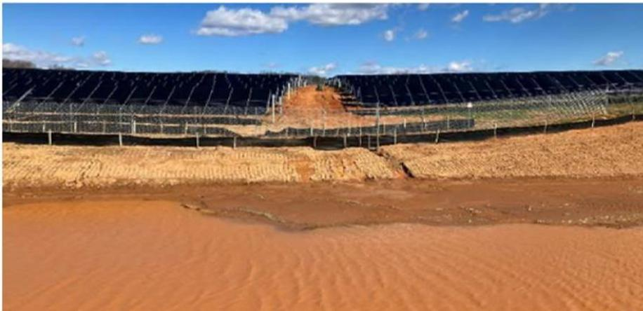
**Figure 6.** Site under active USS development in Virginia before mandatory stabilization and revegetation within 7 days of achieving Final Grade. Final Grade is normally achieved before solar panel installation - but DEQ often sees this requirement ignored resulting in the conditions shown in this photograph.
