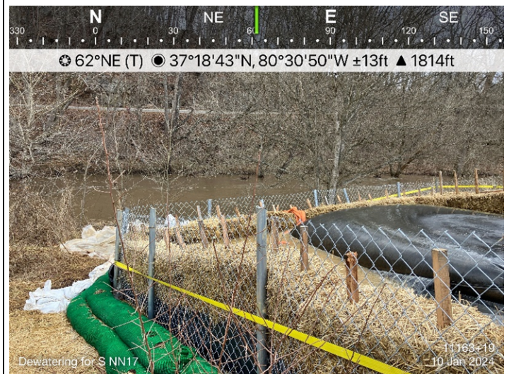
Figure 4: Dewatering structure for S-NN17.
