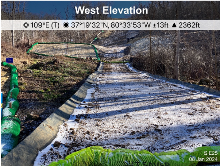
Figure 1: Designated crossing S-E25, ECD's are in place.
