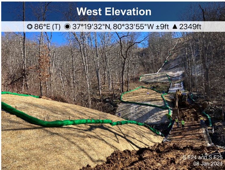
Figure 3: Designated crossing S-E24, ECD's were being maintained.
