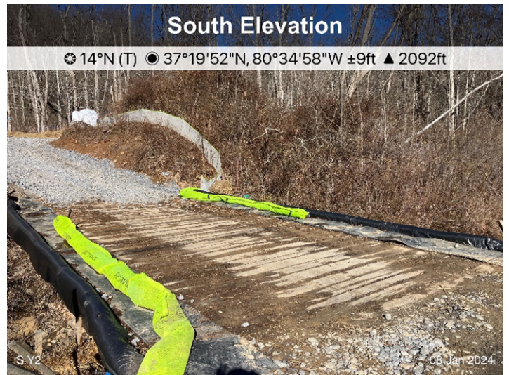
Figure 2: Designated crossing S-Y2. ECD's are in place for active construction.
