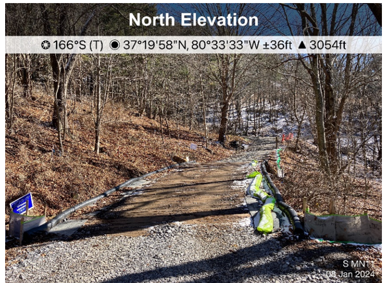
Figure 4: Designated crossing S-MN11, ECD's are in place for active construction.
