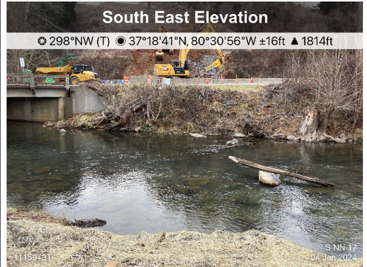
Figure 2: Designated crossing S-NN17. ECD's are in place.
