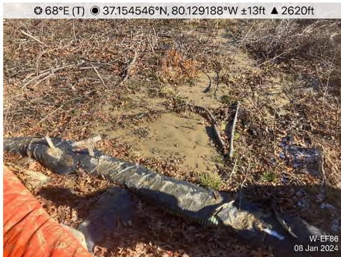
**Figure 4: STA 12869+00** – Sinking matting on equipment bridge is causing ‘pumping’ during use. This ‘pumping’ is causing sediment to inadvertently be pushed from under the matting into the wetland.
