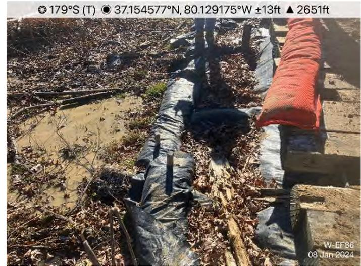
**Figure 3: STA 12869+00** – Sinking matting on equipment bridge is causing ‘pumping’ during use. This ‘pumping’ is causing sediment to inadvertently be pushed from under the matting into the wetland.
