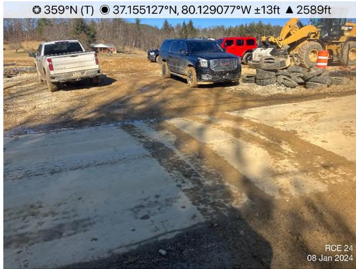
**Figure 2: STA 12869+00** – Sinking matting on equipment bridge is causing ‘pumping’ during use. This ‘pumping’ is causing sediment to inadvertently be pushed under the matting into the wetland.
