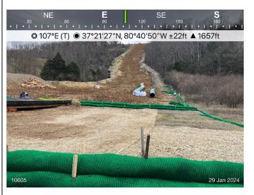
Figure 3: Sta 10710, ECD's are in place.
