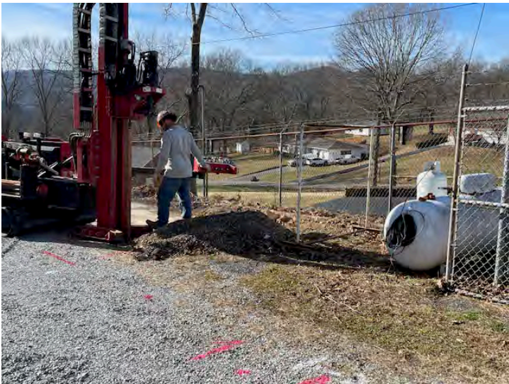
15. Boring B-5 to the north of the UST basin (12/22/2023)
