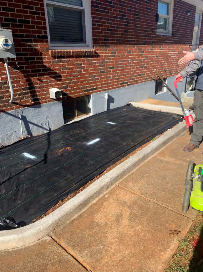
9. Suspected location of heating oil UST at 1556 Coopers Cove Road (12/15/2023)
