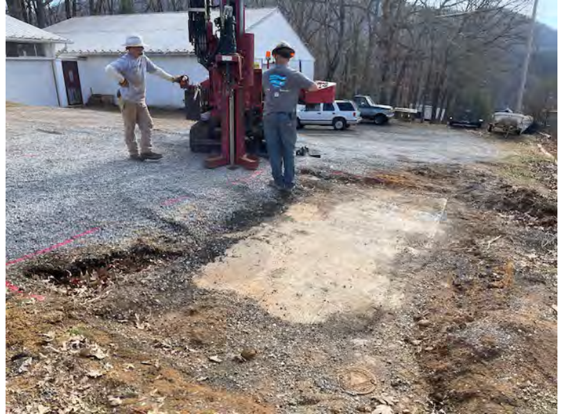
18. Boring B-8 located to the southeast of the UST basin (12/22/2023)
