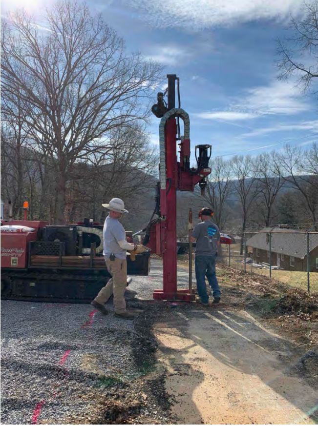
17. Boring B-7 located to the southwest of the UST basin (12/22/2023)
