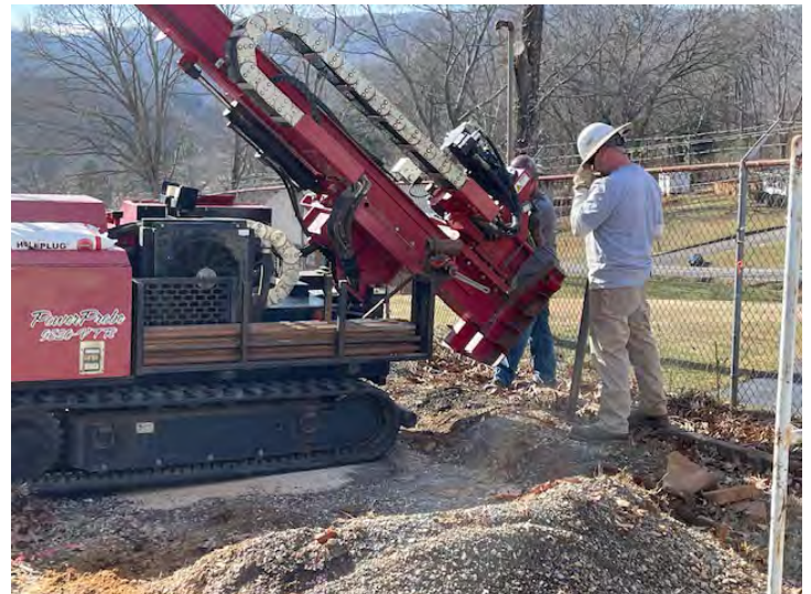
16. Boring B-6 to the west of the UST basin (12/22/2023)
