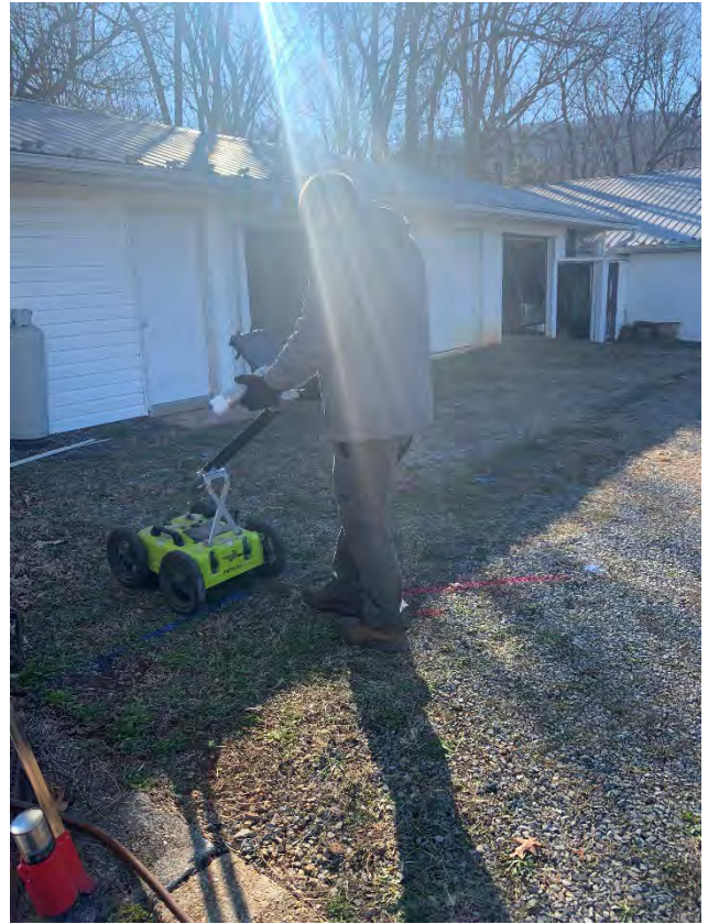
6. Ground penetrating radar and private utility locating (12/15/2023)
