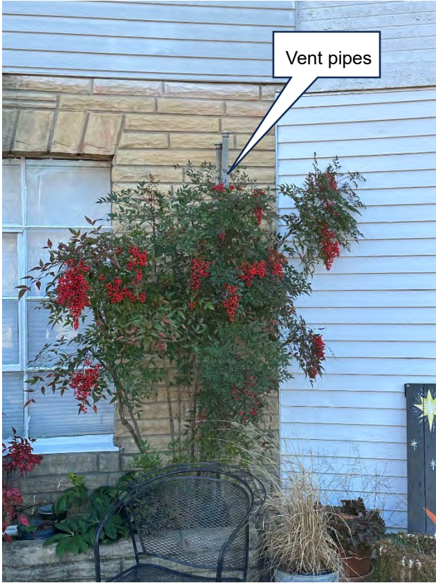
5. Vent pipes noted at 1430 Coopers Cove Road (12/15/2023)
