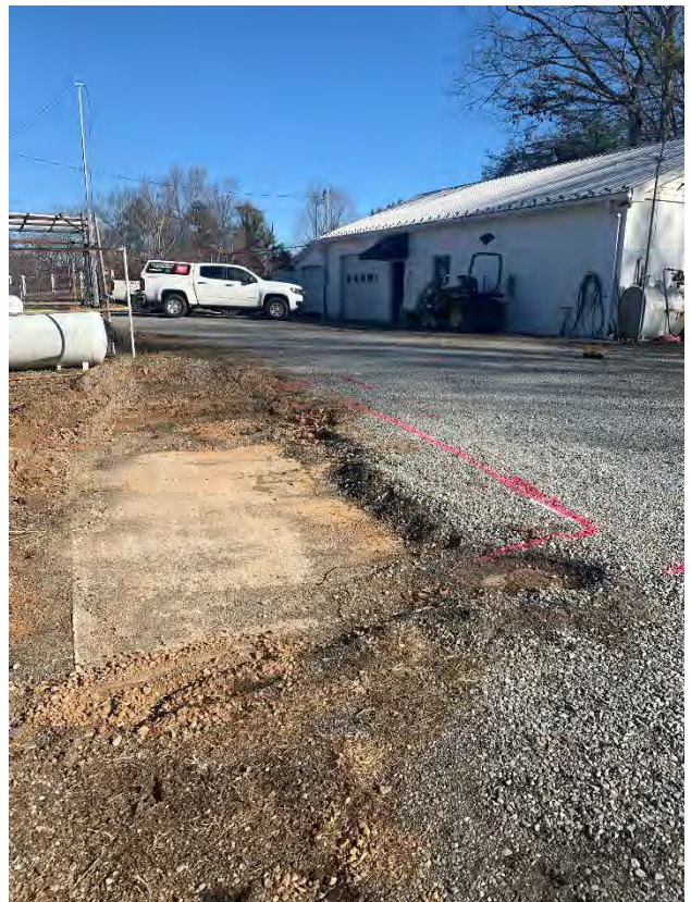
8. UST basin uncovered at 1640 Coopers Cove Road (12/15/2023)
