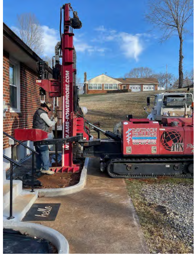
10. Soil boring B-1 near heating oil UST at 1556 Coopers Cove Road (12/22/2023)
