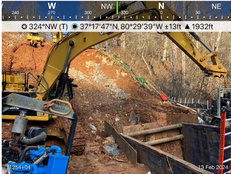
**Figure 2:** ATWS 1370, ESC devices were in place along with dewatering tanks.
