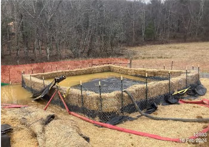
Figure 3: STA 12893+00 – Dewatering structure #2 installed and functioning properly.
