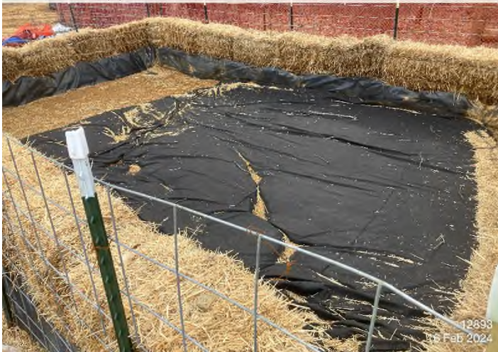
Figure 3: STA 12893+00 – Dewatering structure #2 installed and functioning properly.
