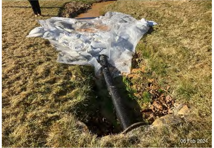
Figure 4: Rt. 42 and Clover Hollow Dr. – CFS check dams installed within stormwater conveyance channel prior to entering Sinking Creek.
