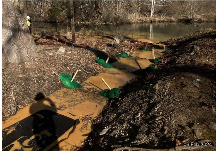
Figure 4: Rt. 42 and Clover Hollow Dr. – CFS check dams installed within stormwater conveyance channel prior to entering Sinking Creek.
