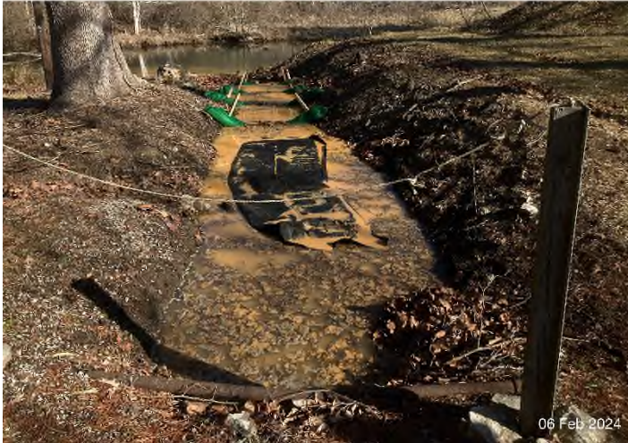
Figure 3: Rt. 42 and Clover Hollow Dr. – North side of Clover Hollow Drive. Flume is connected to sediment bag prior to entering stormwater channel.
