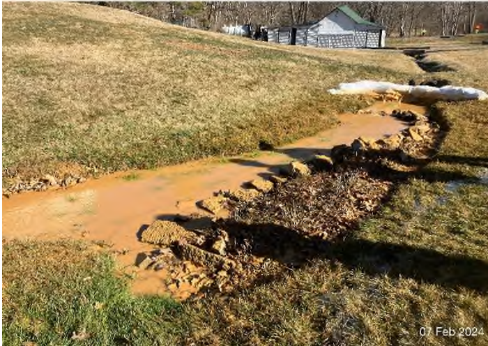
Figure 3: Rt. 42 and Clover Hollow Dr. – Flume pipe discharges to sediment filter and is further treated by a rock check dam and several CFS check dams prior to entering Sinking Creek.
