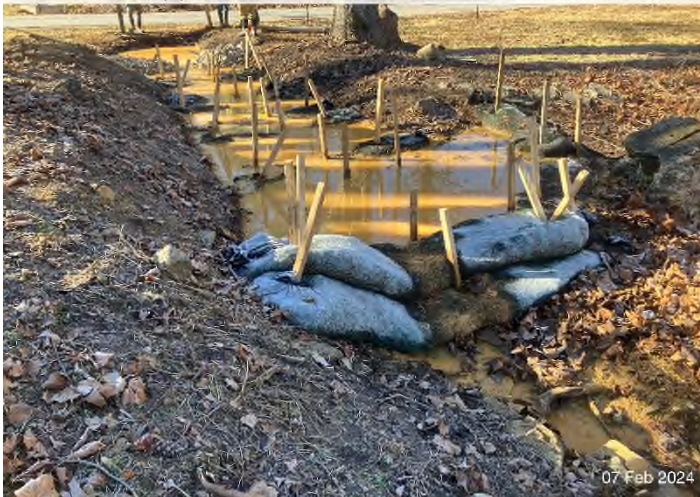
Figure 3: Rt. 42 and Clover Hollow Dr. – Flume pipe discharges to sediment filter and is further treated by a rock check dam and several CFS check dams prior to entering Sinking Creek.
