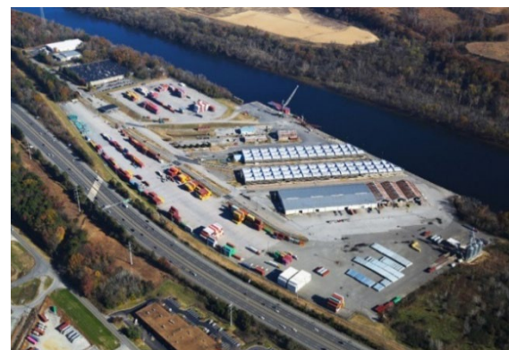
Figure 14. Richmond Marine Terminal
