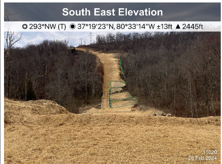
Figure 4: Sta 11020, area is stabilized and ESC is in place.
