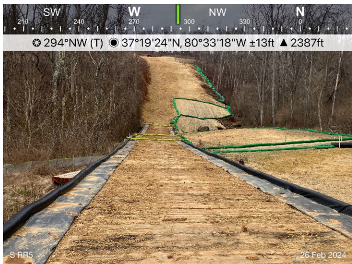
Figure 3: Designated stream S-RR5, ESC is in place.
