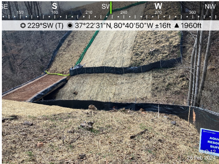
Figure 1: Designated stream S-Q12, ESC is in place.
