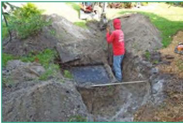
Septic System Repair
