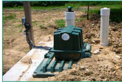
Alternative On-site Sewage Disposal System
