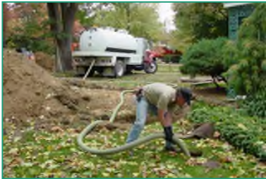
Septic System Pump out
