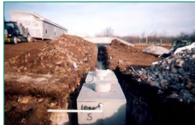
Conventional Septic System Replacement
