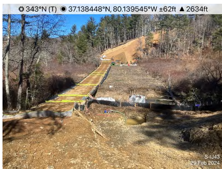
Figure 7: Stream S-IJ43/Wetland W-IJ36 – Looking north at active bore site for Mill Creek and associated wetland. Controls in place and functioning properly.
