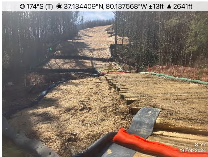
Figure 7: Stream S-IJ43/Wetland W-IJ36 – Looking north at active bore site for Mill Creek and associated wetland. Controls in place and functioning properly.
