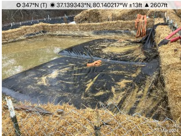
Figure 7: STA 12938+00 – Dewatering structure for boring operation.
