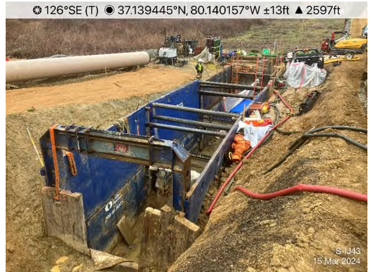
Figure 8: STA 12938+00 – Bore pit entrance for S-IJ43 and W-IJ36.
