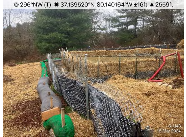
Figure 6: STA 12938+00 – Dewatering structure for boring operation at S-IJ43 and W-IJ36.
