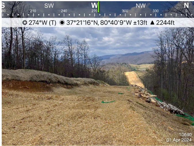
Figure 1: Sta 10640, ESC and stabilization in place.
