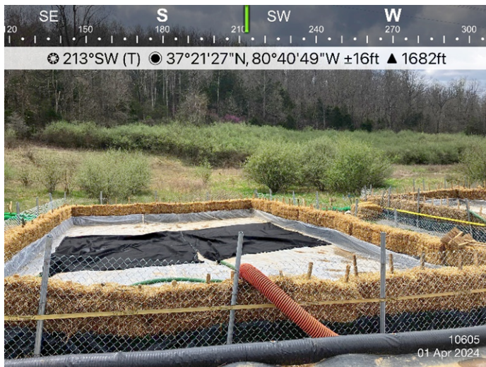
Figure 3: Sta 10605, dewatering structures in place.
