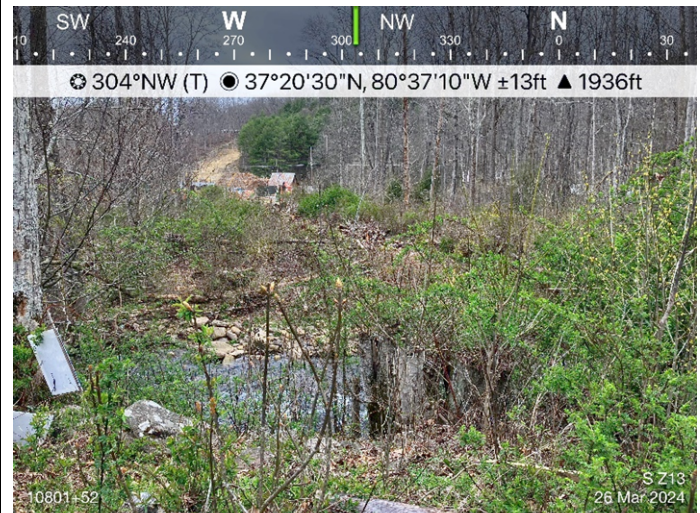
Figure 4: Designated crossing S-Z13, ESC devices in place.
