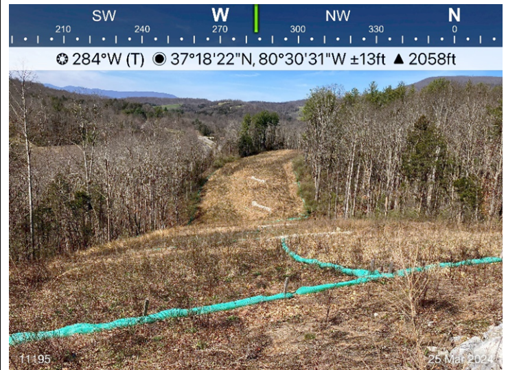
Figure 4: Sta 11195, ESC and permanent style waterbars are in place.
