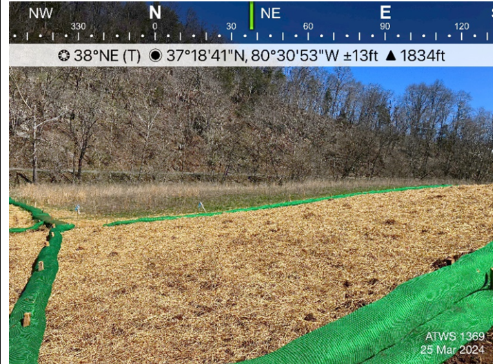
Figure 2: ATWS 1369, stabilization and ESC are in place.
