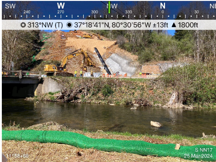
Figure 1: Designated crossing S-NN17, stabilization and ESC are in place.
