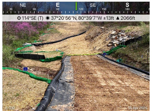
Figure 4: Designated crossing S-G32, ESC in place.
