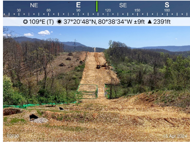
Figure 2: Sta 10730, ESC and stabilization in place.
