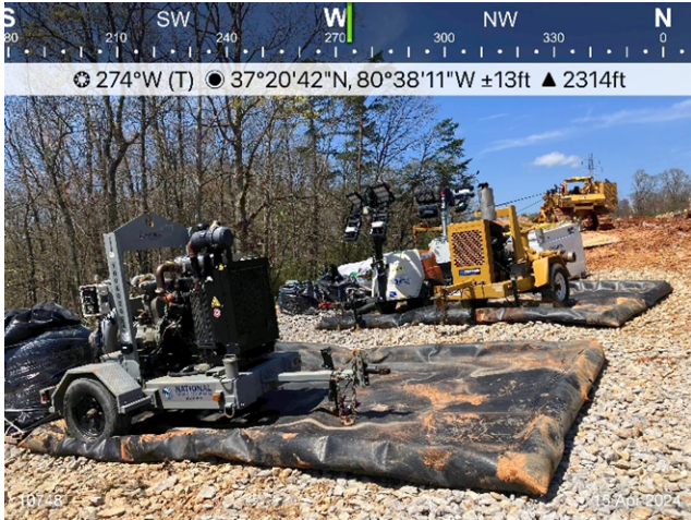
Figure 1: Sta 10748, 2 nd containment in place.
