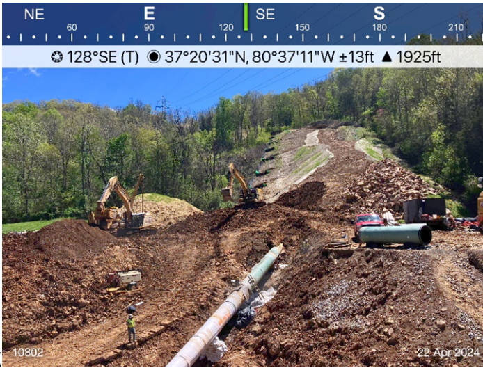
Figure 1: Sta 10802, bore site for designated crossing S-Z13.
