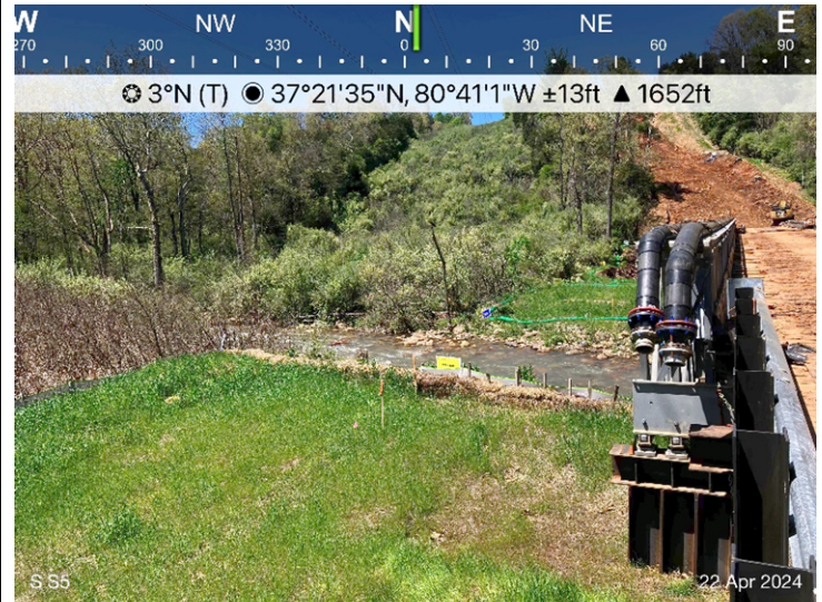
Figure 2: Designated crossing S-S5, ESC is in place.
