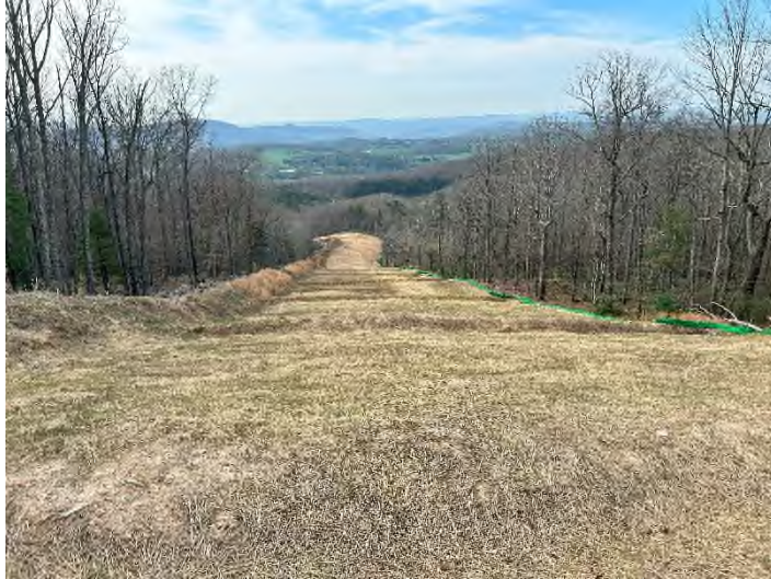
Figure 1: STA 11674+00 – Controls in place and functioning properly.
