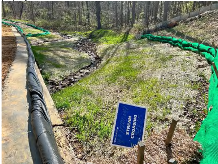
Figure 3: STA 11740+00 – Controls in place and functioning properly.
