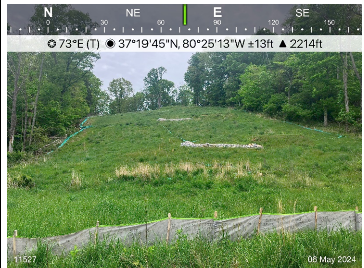
Figure 4: Sta 11527, ESC in place.
