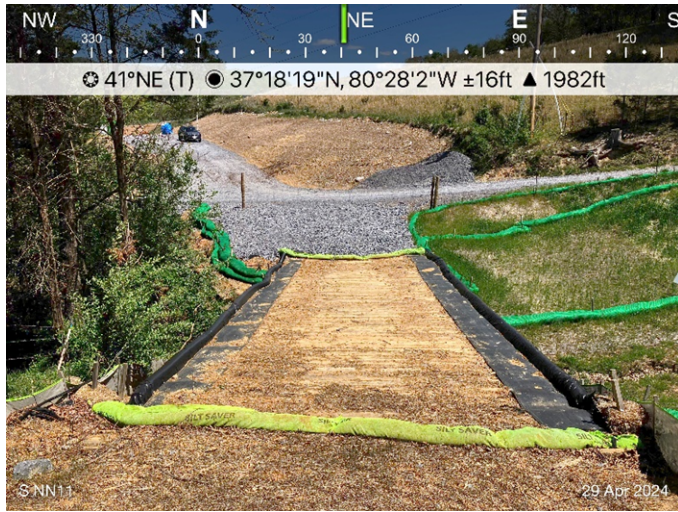
Figure 1: Designated crossing S-NN11, ESC is in place.
