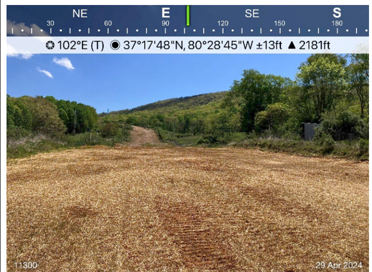
Figure 4: Sta 11300, ESC in place.
