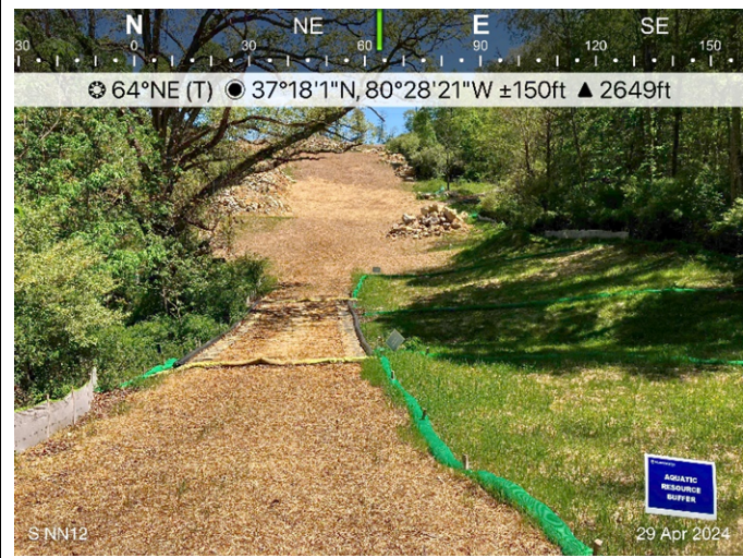
Figure 2: Designated crossing S-NN12, ESC is in place.
