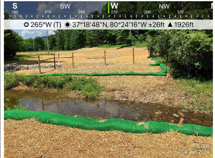
Figure 2: Designated crossing S-006, ESC is in place.
