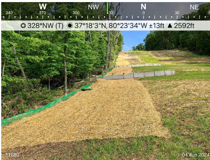
Figure 3: Sta 11680, ESC is in place.
