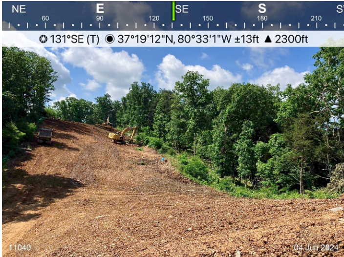
Figure 1: Sta 11040, final grading is being constructed.
