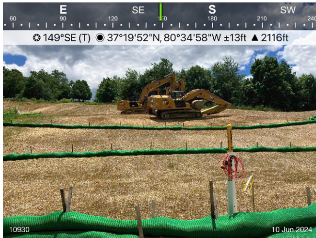
Figure 3: Sta 10930, ESC is in place.
