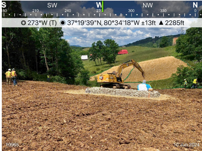
Figure 1: Sta 10965, final grading is being constructed.
