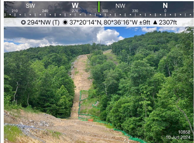
Figure 4: Sta 10858, ESC is in place.
