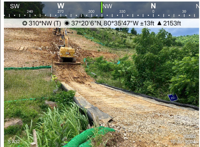
Figure 2: Designated crossing S-A32, ESC is in place for active construction.
