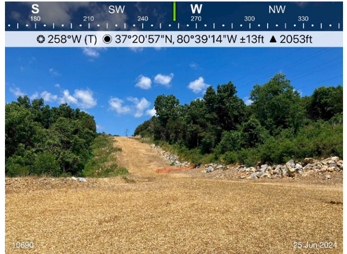
Figure 4: Sta 10690, ESC is in place.
