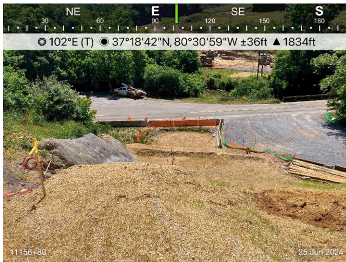
Figure 3: Sta 1156+80, ESC is in place.
