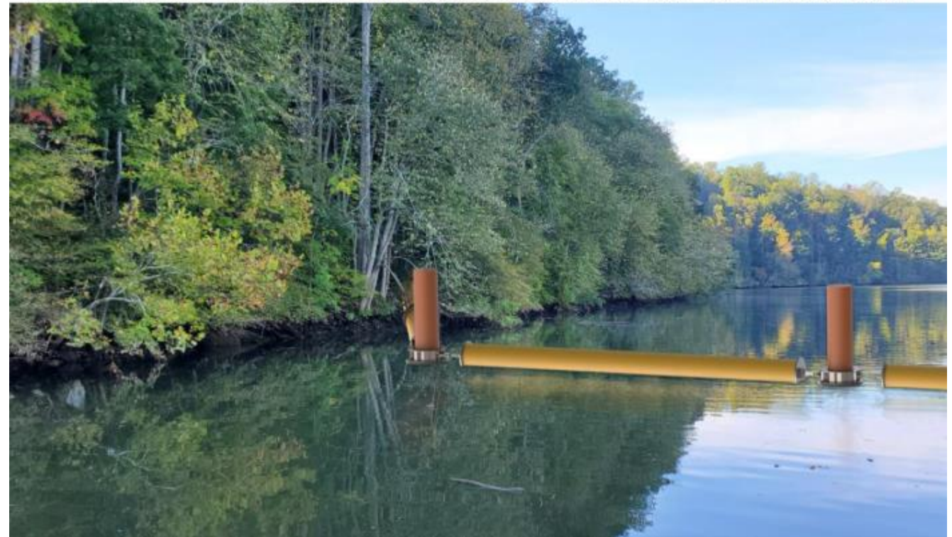
BOOM ANCHOR POINT ALONG SOUTHERN BANK OF LEESVILLE LAKE - LOOKING UPSTREAM
