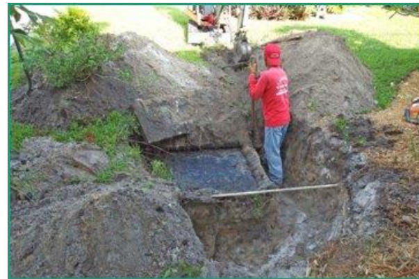
Septic System Repair
