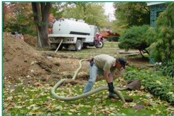
Septic System Pump out
