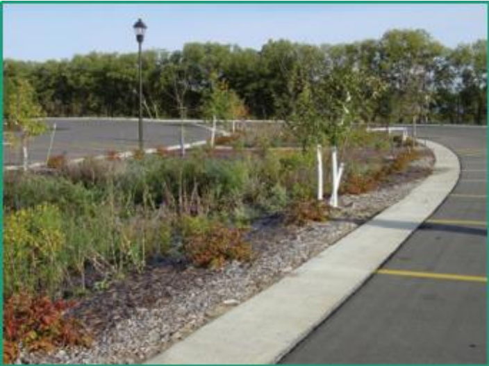
Bio Retention (Rain Garden)
