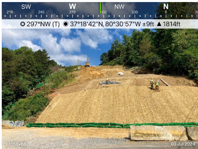
Figure 3: Sta 11158+68, ESC is in place.
