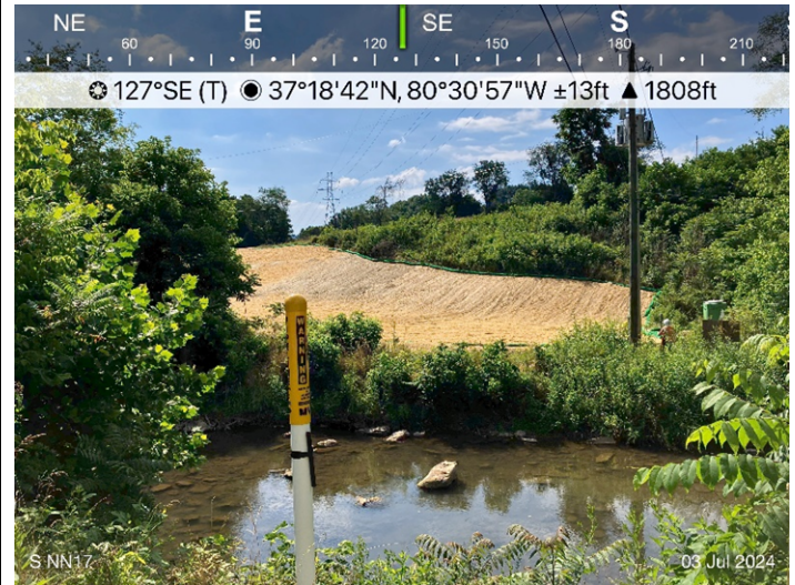
Figure 2: Designated crossing S-NN17, ESC is in place.
