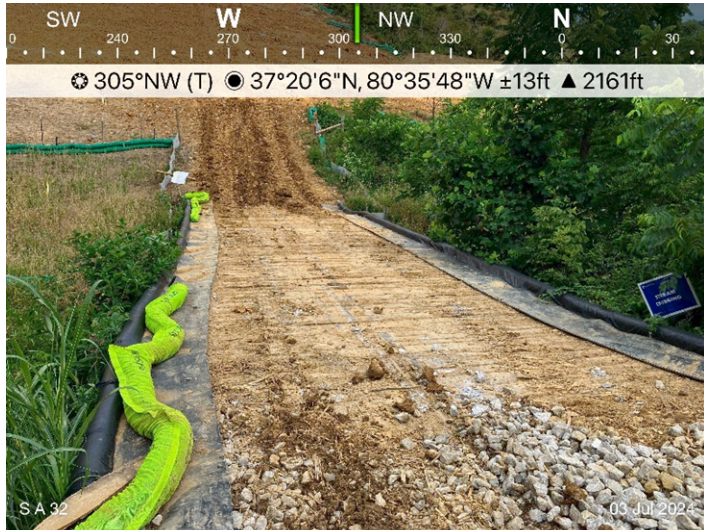
Figure 1: Designated crossing S-A32, ESC is in place for active construction.
