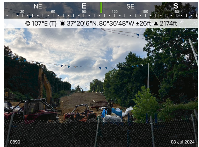
Figure 4: Sta 10890, permanent waterbars are being constructed and ESC is in place.
