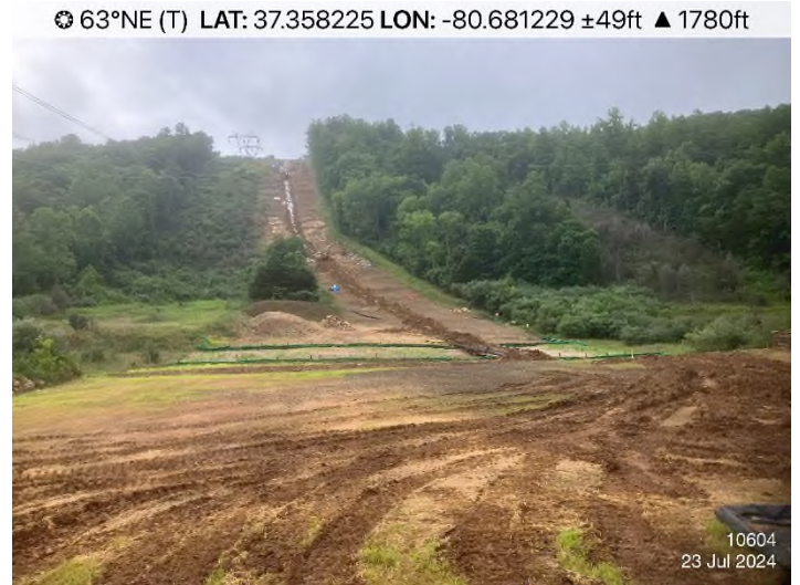
Fig. 2 STA 10604+00: Controls in place and functioning properly.
