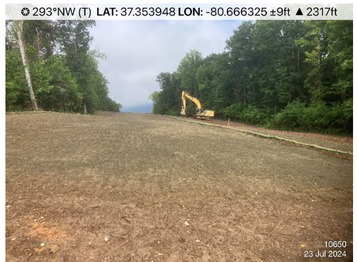
Fig. 4 STA 10650+00: Controls in place and functioning properly.
