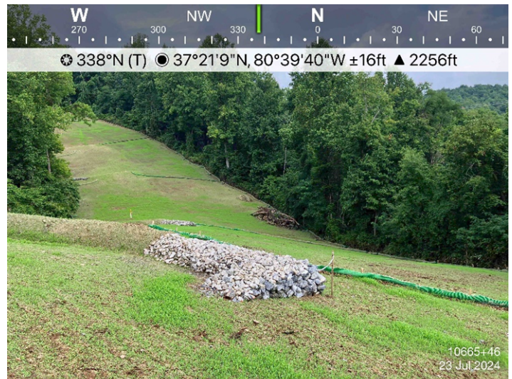
Fig. 4 Description: Sta 10665+46, permanent waterbars in place.
