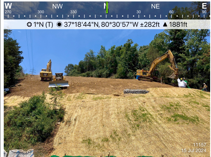
Figure 4: Sta 11157, permanent waterbars are being constructed and ESC is in place.
