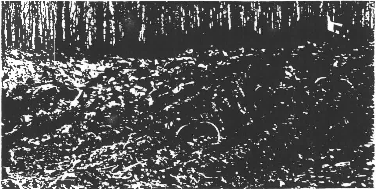
The area fill method is being used at this Virginia landfill.
