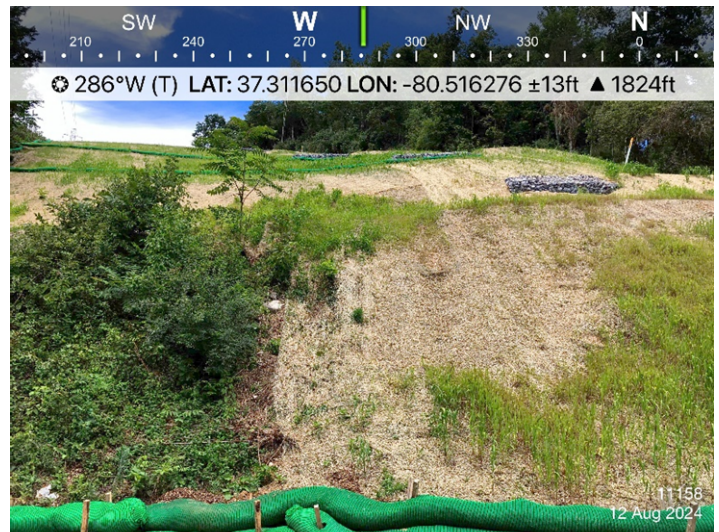
Fig. 4 Description: Sta 11158+64, permanent waterbars in place.
