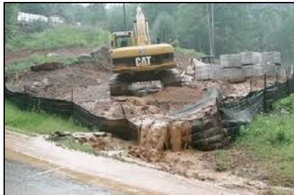
Figures 12 and 13: Construction site erosion and runoff
