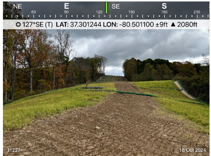
Fig. 2 Description: Sta 11227, ESC is in place.
