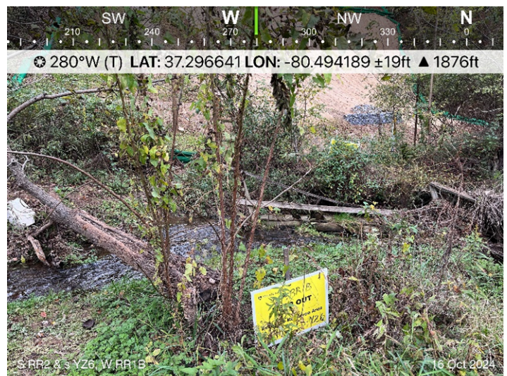
Fig. 4 Description: Designated crossing S-YZ6, SRR2, & W-RR1B ESC is in place.
