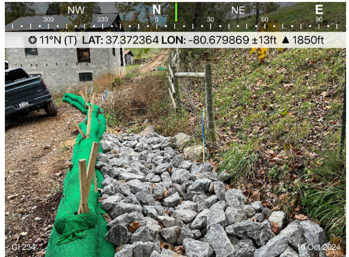
Fig. 4 Description: GI 234, ESC is in place.
