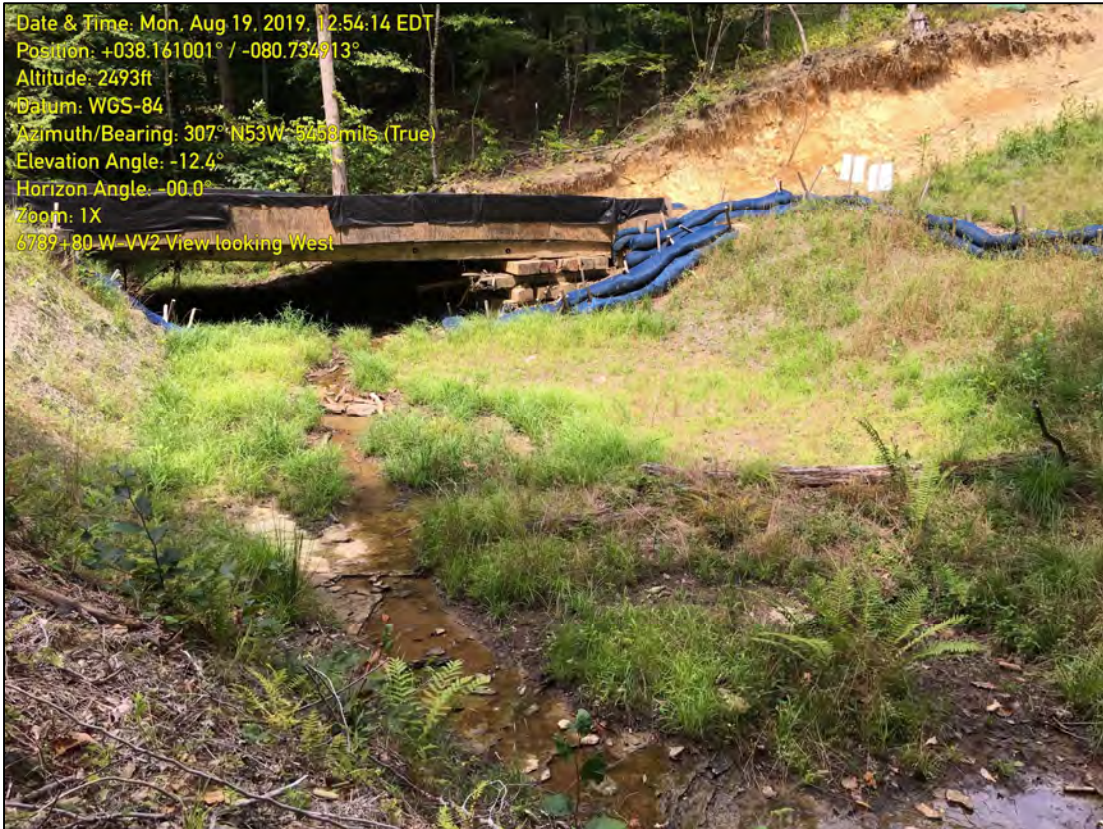
Photo illustrates the restored stream S-VV1 and wetland W-VV2 (August 2019)
