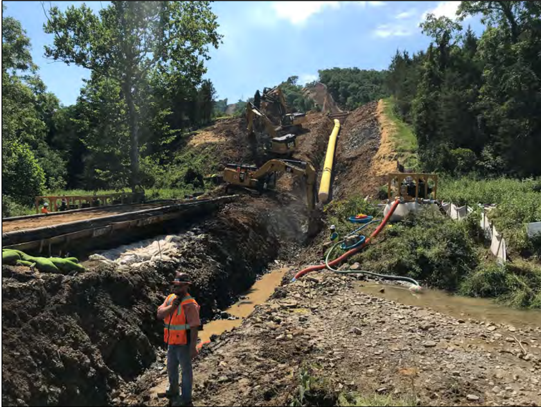
Photo illustrates the active construction of Northfork Roanoke River crossing (July, 2018)
