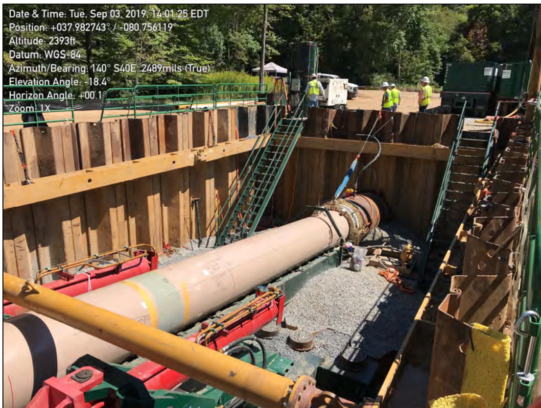
Both photo illustrate Direct Pipe drill rig for the Meadow River crossing.
