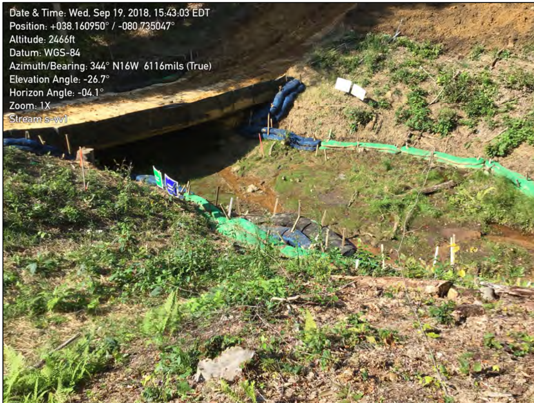
Photo illustrates the preconstruction conditions of stream S-VV1 and wetland w-VV2.
