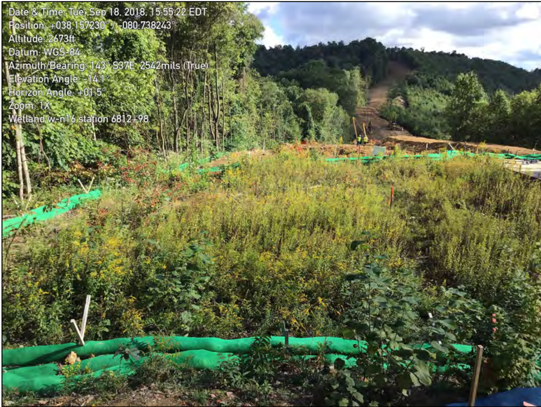
Photo illustrates the preconstruction conditions of wetland W-N16 (September 2018)
