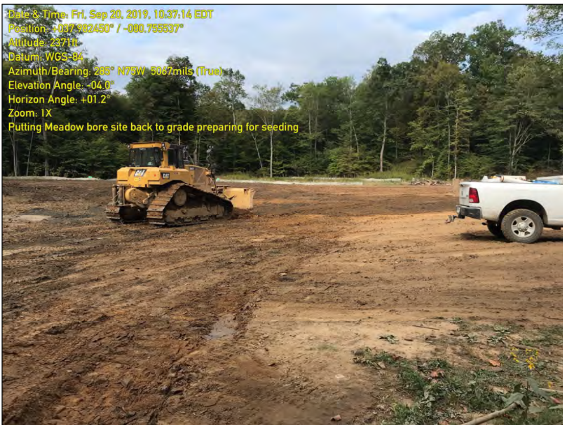
Photo illustrates the final grading of the bore prior to seeding.
