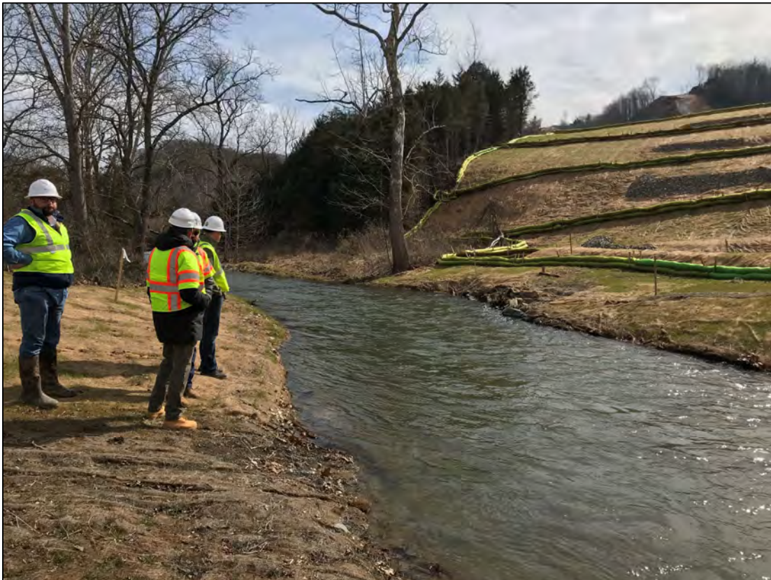
Photo illustrates the restored crossing of Northfork Roanoke River crossing (February, 2019)
