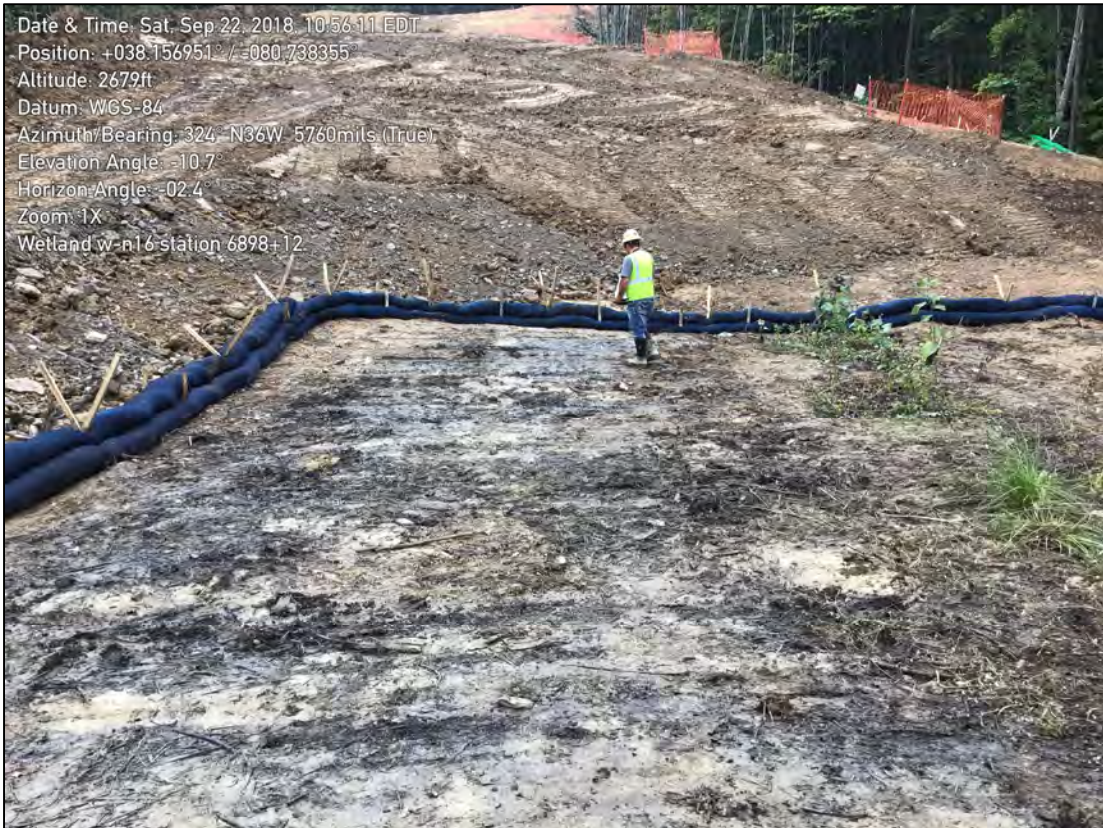
Photo illustrates wetland W-N16 immediately following installation and backfill (September 2018).
