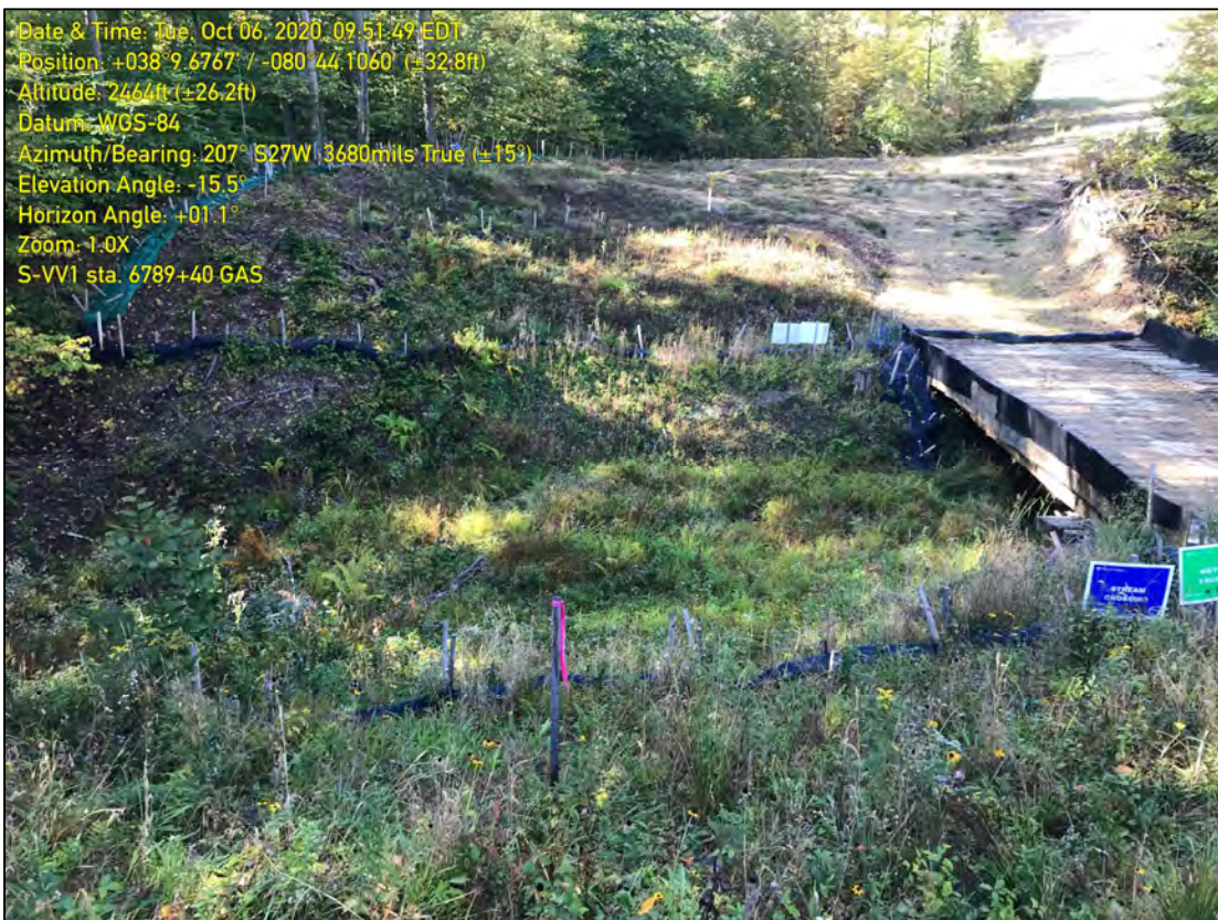
Photo illustrates the restored stream S-VV1 and wetland W-VV2 (October 2020)
