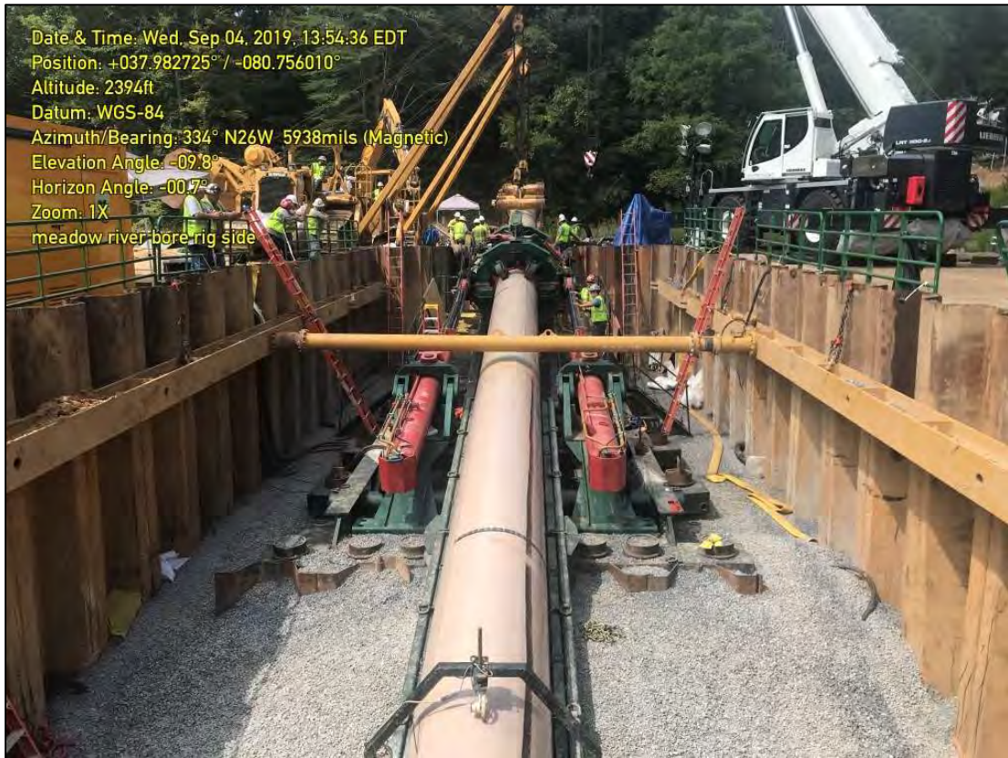
Both photo illustrate Direct Pipe drill rig for the Meadow River crossing.
