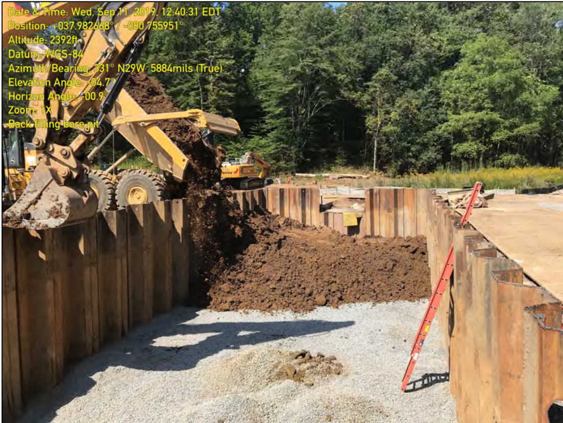
Photo illustrates the backfilling of the Meadow River bore pit.
