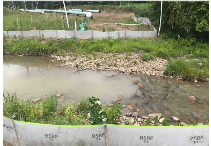
Figure 4: Stream S-006 – Controls in place and functioning properly around Craig Creek crossing.
