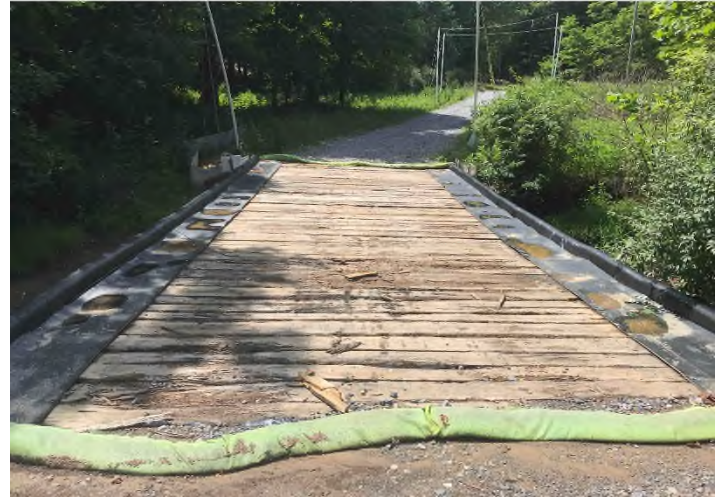
Figure 4: Stream S-006 – Controls in place and functioning properly around Craig Creek crossing.
