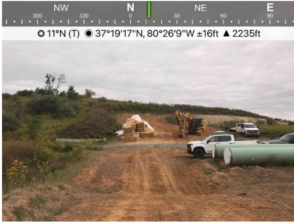
Figure 1: MVP E&S crews working near MP217.1
