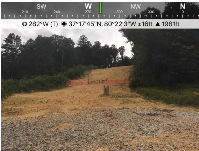
Figure 3: Gate installed near MLV 26 and area has been recently re stabilized.
