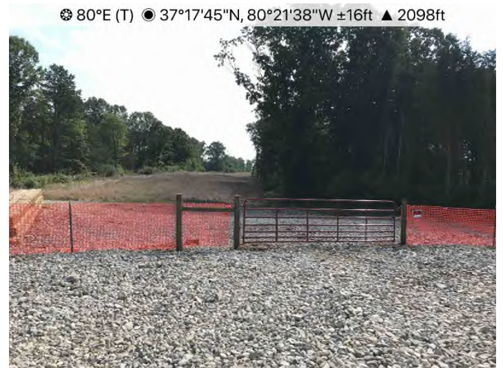
Figure 4: STA 11792+00 – Fencing and gate installed.
