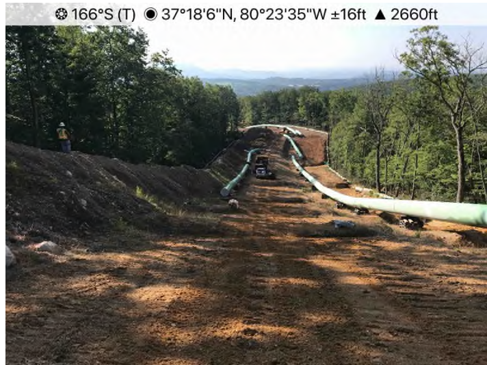
Figure 3: STA 11765+00 – Fencing and gate installed. Crews actively stabilizing with seed and straw.
