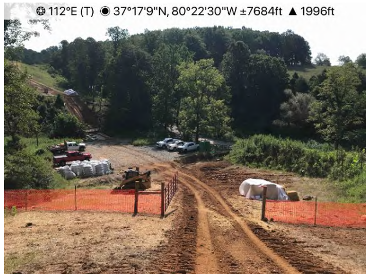
Figure 3: STA 11765+00 – Fencing and gate installed. Crews actively stabilizing with seed and straw.
