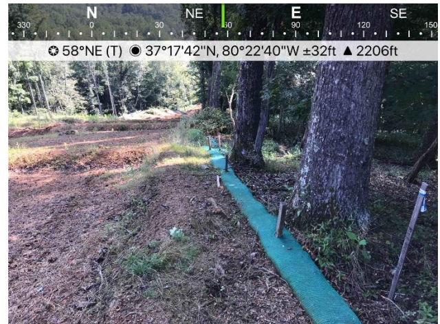
Figure 4: Near St11734 ECD's are in place.
