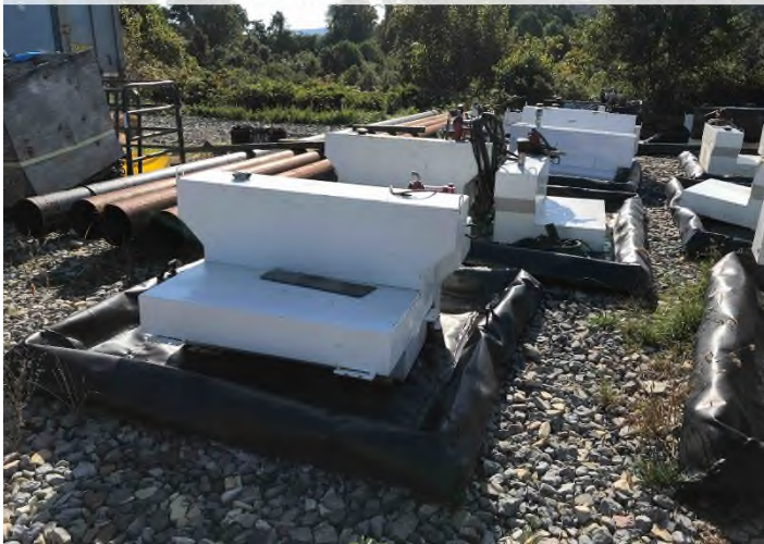
Figure 3: Laydown Yard 026 – Secondary containment in place and functioning properly.
