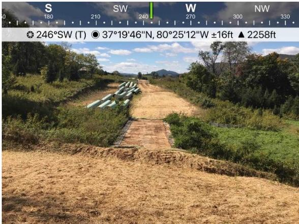
Figure 2: Designated stream crossing S-Y2, ECD's are in place.
