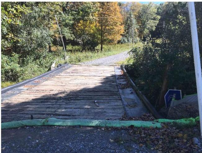
Figure 4: Designated stream crossing S-006, ECD's are in place
