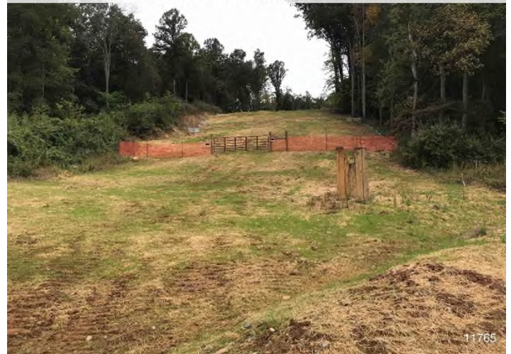
Figure 4: STA 11765+00 – Controls in place and functioning properly. Area stabilized with straw.
