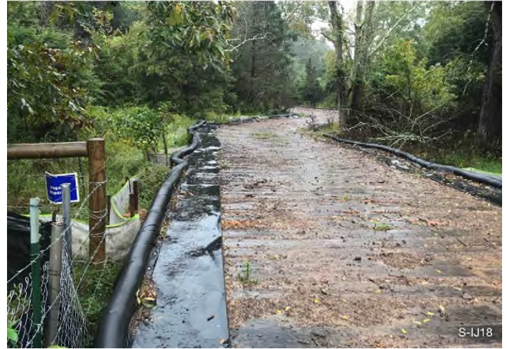
Figure 4: STA 11765+00 – Controls in place and functioning properly. Area stabilized with straw.
