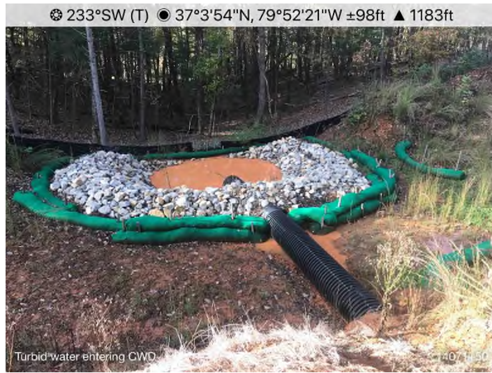
Figure 3: STA 14083+00 – CFS maintenance needed.
