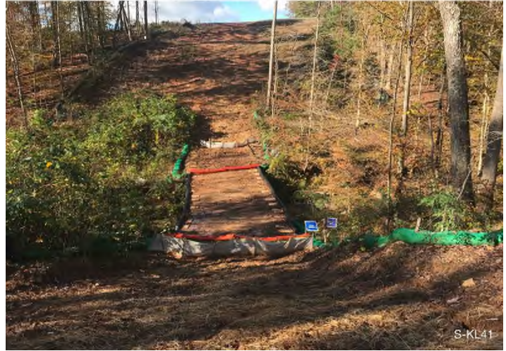
Figure 6: Stream S-KL41 – Unnamed trib. to Blackwater River crossing looking west at crossing. Controls in place and area stabilized with straw.
