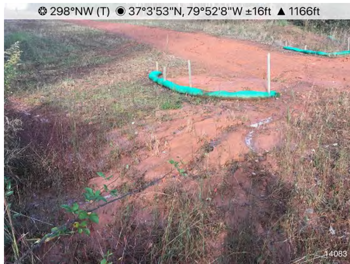
Figure 3: STA 14083+00 – CFS maintenance needed.
