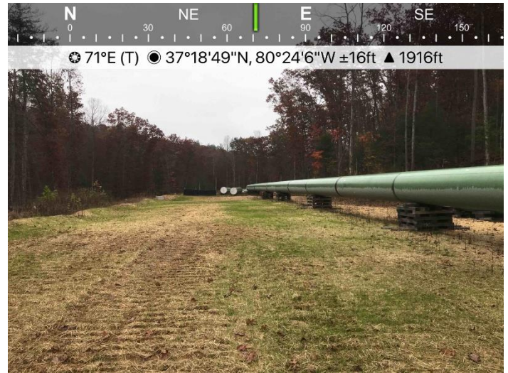
- Figure 4: Near MP 219.5 area is stabilized and ECD's are in place.
