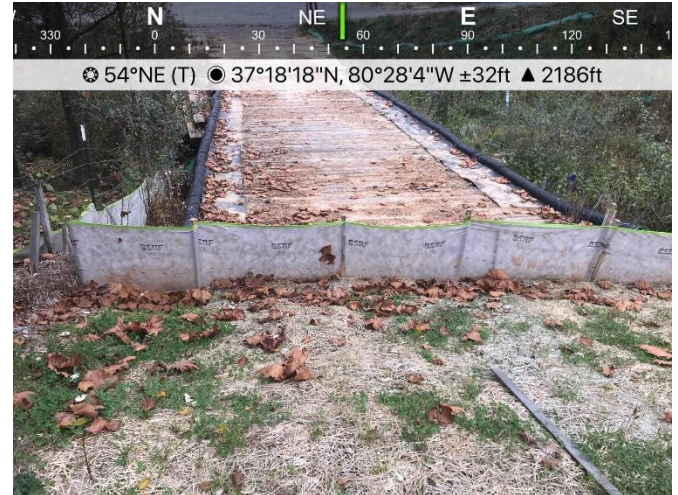
Figure 4: Designated stream crossing S-NN11, ECD's are in place.
