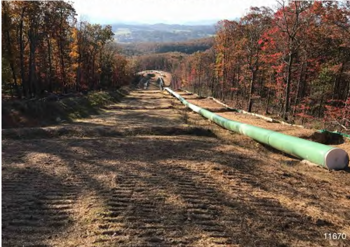
Figure 1: Stream S-MN22 – Controls in place and functioning properly around stream S-MN22 crossing.
