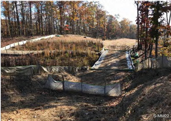
Figure 1: Stream S-MN22 – Controls in place and functioning properly around stream S-MN22 crossing.
